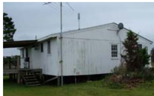
FIGURE 185B. The same view in 2006. Note the addition to the building along its rear facade, the removal of the screened porch, replacement of the siding, and the addition of a deck.
