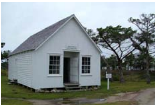
FIGURE 187B. The same view today. Changes since the 1930s include the loss of the addition, and removal of the porch and overhang. The vent pipe in the rear is also gone. The side door indicates the former connection between this building and the missing addition.
