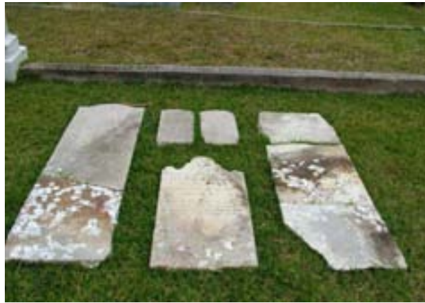
FIGURE 204. Biological growth and sugaring have affected these grave markers.
