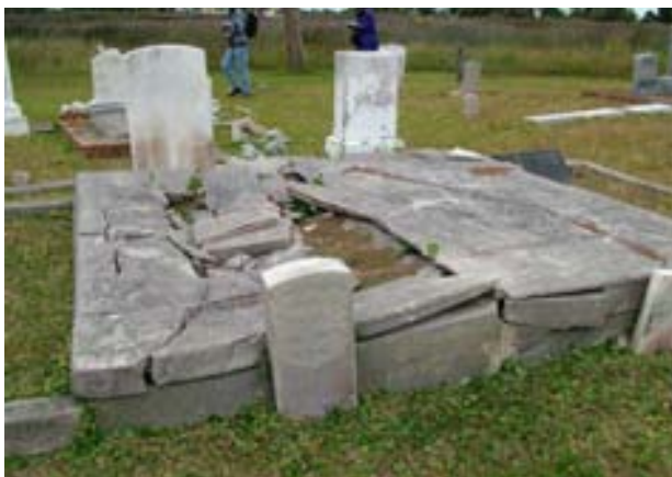
FIGURE 208. Cracking and displacement of concrete vaults can allow water to pond, accelerating deterioration of the feature.
