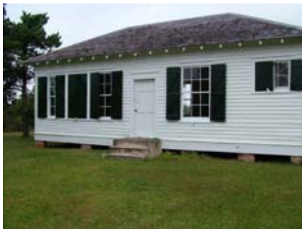
FIGURE 168B. The same view in 2006. Note the loss of the brick landing and walk, changes in paint color on the door and shutters, the reconfiguring and reshingling of the roof, and the loss of foundation plantings since 1969.
