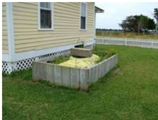
FIGURE 41. Above-ground septic systems are typically used for wastewater treatment and management in association with most buildings.
