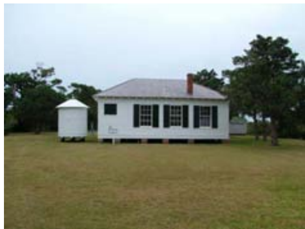
FIGURE 45. The original entrance to the schoolhouse was at the end wall where the cistern is now located. This former entrance was closed up when the building was converted to living quarters circa 1940s.
