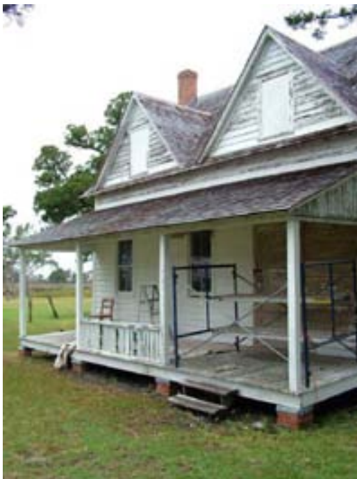
FIGURE 178B. The same view in 2006. Note the replacement of the central dormer with two dormers and alteration of the porch posts and railing. Woodwork beneath the porch is no longer present.
