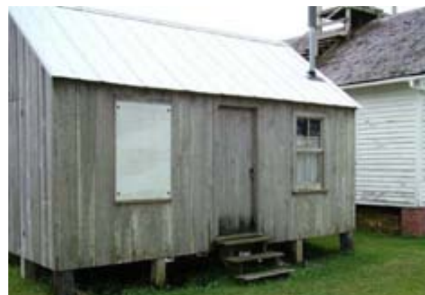
FIGURE 192B. The same shed in 2006. Changes visible between the photographs includes the boarded window, different cladding of the shed, the addition of a vent pipe, replacement of the door, addition of wooden steps, lack of paint, and the addition of the widow's walk to the roof of the adjacent Carl Dixon House.
