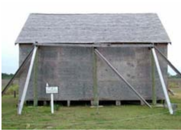
FIGURE 186B. The George Dixon House in 2006 is mothballed following severe hurricane damage.
