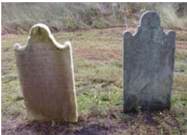
FIGURE 207. General soiling affects many of the markers in the district, such as the two seamen's grave markers. Evidence of rising damp is also visible here.
