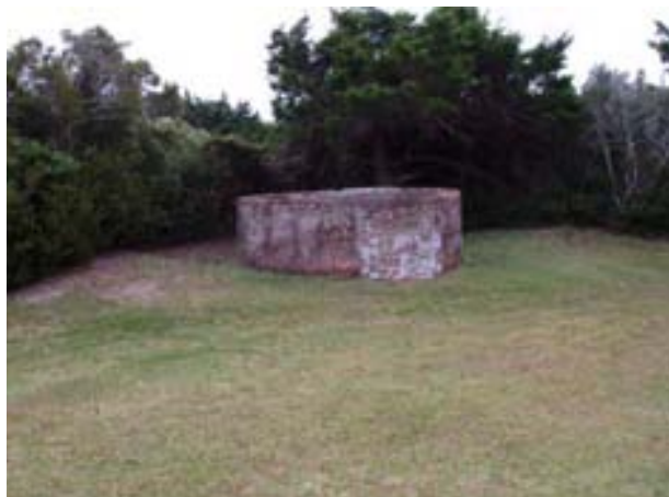
FIGURE 40. Cisterns like the U.S. Marine Hospital structure shown here are used to store rainwater on the island and are the primary source of fresh water.
