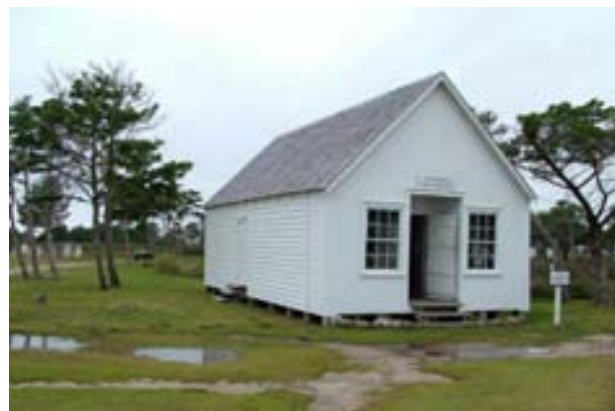
FIGURE 188B. The same view today. Changes since the 1930s include the loss of the addition, and removal of the porch and overhang. The vent pipe in the rear is also gone.
