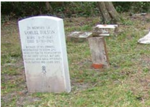
FIGURE 209. Rising damp has discolored the Samuel Tolson marker.
