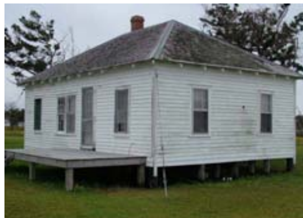
FIGURE 184B. The same view today. Note the loss of the roof overhang associated with the porch and the wood stair and landing along the side/rear of the house. The vegetation is now mown cool-season grass, whereas the earlier view suggests native warm-season grasses were present previously. Cabling is currently stabilizing the structure.
