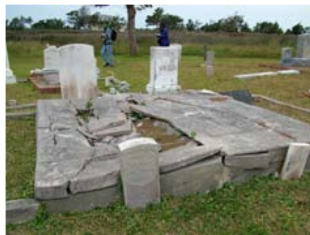
FIGURE 131. The condition of some of the concrete vault covers in the Community Cemetery is poor.
